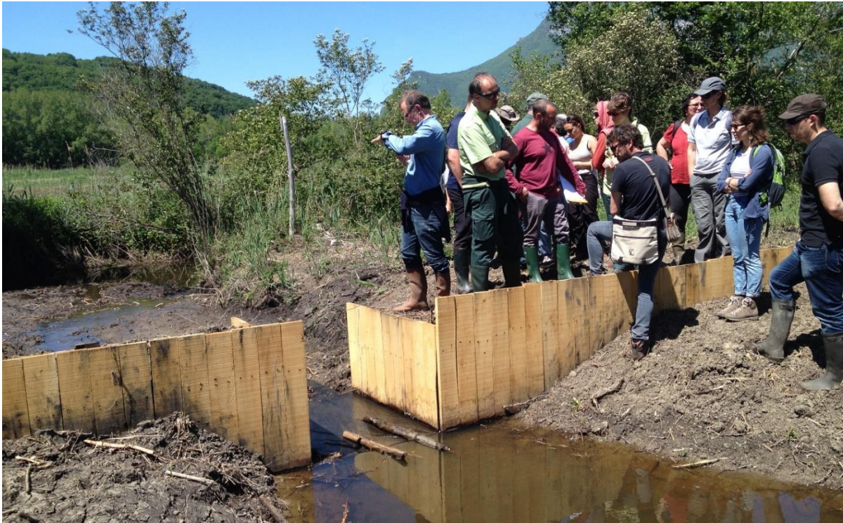
Fig. 8: “Rewetting” measures in the forested part of the Marais de Chautagne. Raising water table for another 80 cm would be necessary for the development of wetland biodiversity and the reduction of greenhouse gas emissions.
