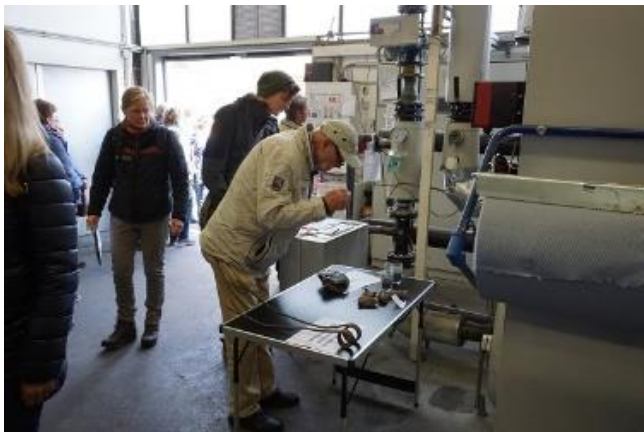
7 Visitors at the heating plant Malchin (Photo: A. Haberl)
